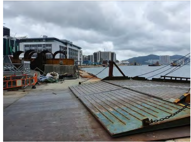
Temporary trench had been installed at the sea front to prevent muddy run-off overflow into the water body during rainstorm.
