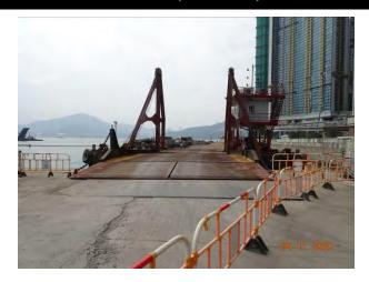
Temporary trench had been installed at the sea front to prevent muddy run-off overflow into the water body during rainstorm.
