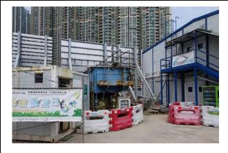
Treatment facilities was installed at site to treat the site generated water prior discharge.
