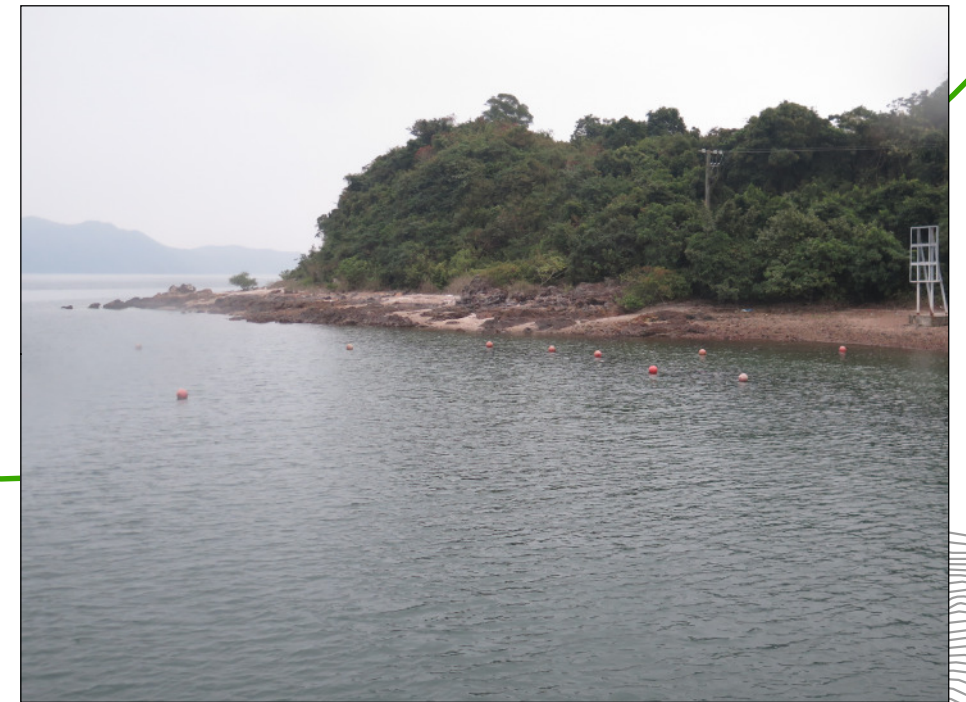
Current Conditions of the Landing Site at Liu Ko Ngam (Photo captured in December 2015)
