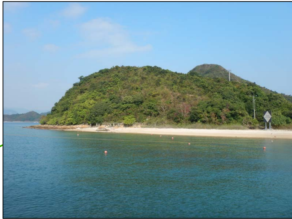
Current Conditions of the Landing Site at Pak Sha Tau Tsui (Photo captured in January 2016)
