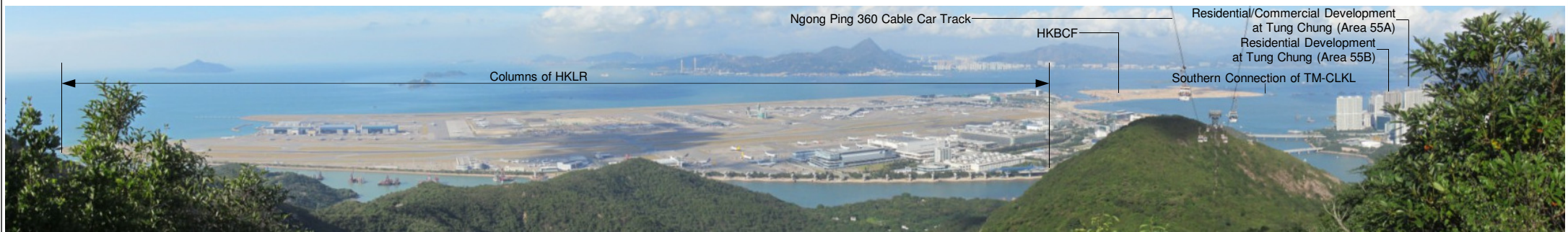
Existing Baseline Conditions in November 2015
