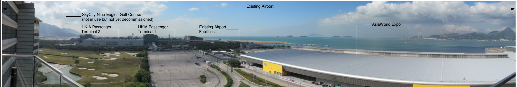
Existing Baseline Conditions in November 2015
