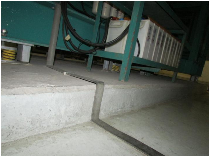
HS1 View 4 - concrete floor condition underneath emergency generators
