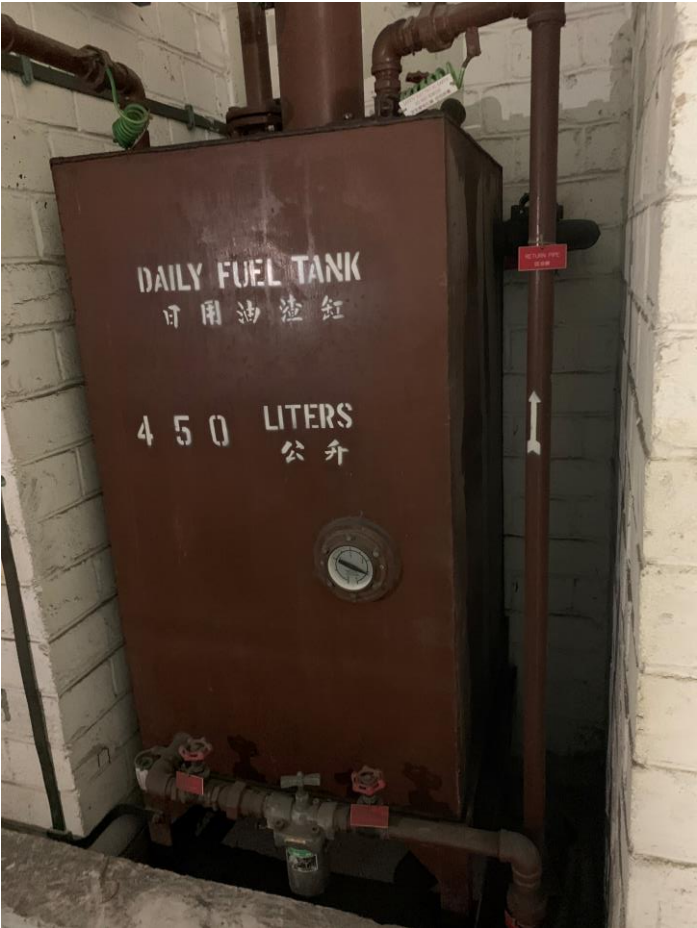
BH7 View 1 - 450 L Above-ground Fuel Tank
