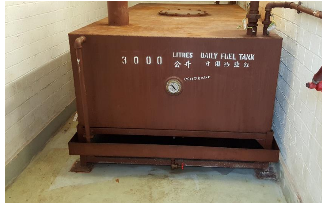
BH9 View 1 - 3000L Above-ground Fuel Tank (BH9)
