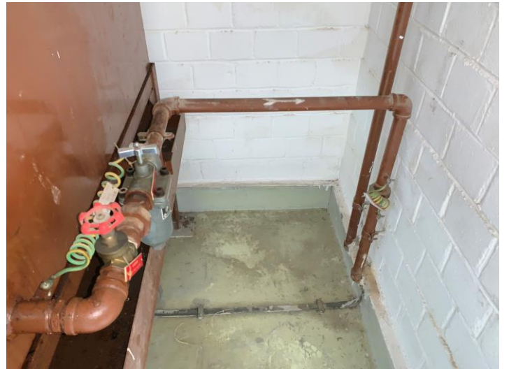
HS4 View 2 - concrete floor condition of fuel tank room with 1,500 L above-ground fuel tank
