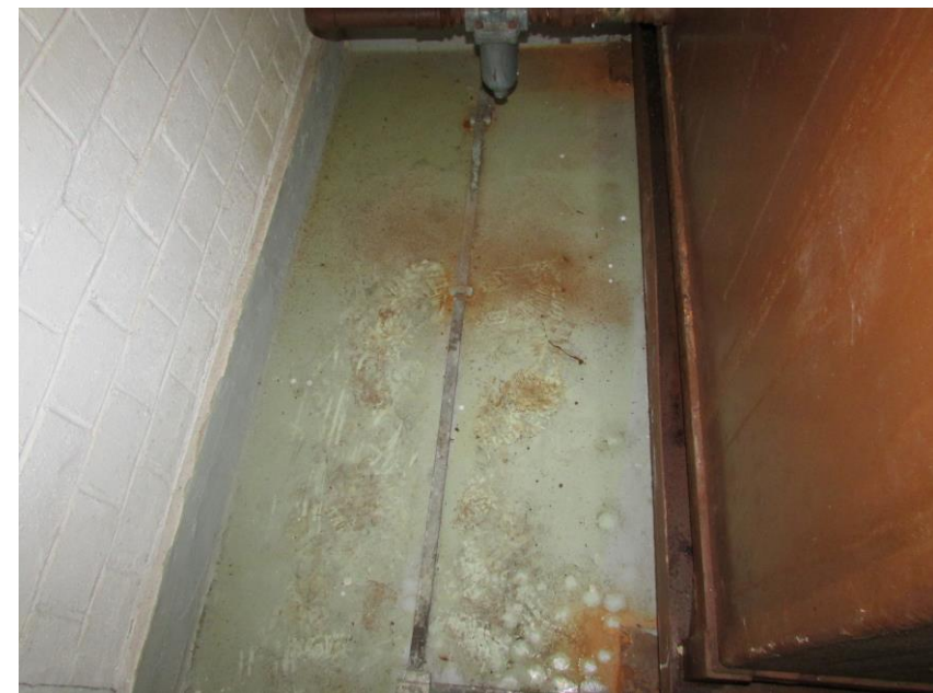
BH9 View 3 - concrete floor condition of fuel tank room with 3000L Above-ground Fuel Tank
