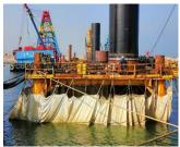
Silt Curtain deployed by Contractor for Piling Activities
