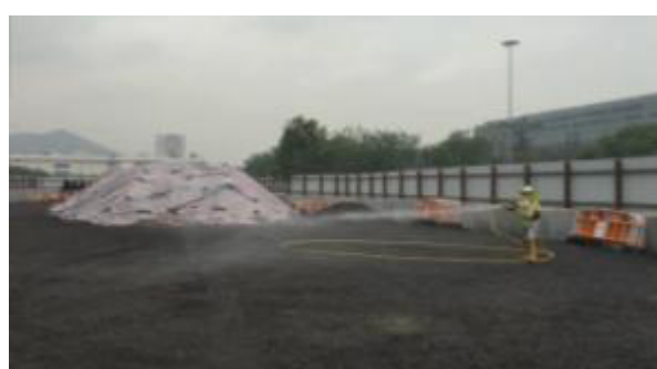
Stockpiling of excavated material at stockpiling area
