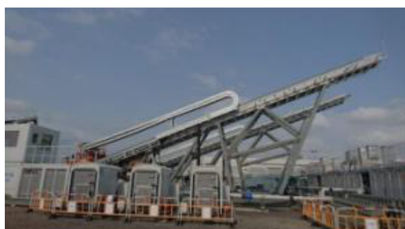
Installation of HDD casing pipe at HDD launching site
