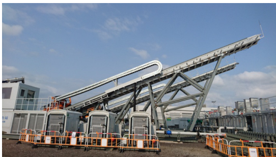
Installation of HDD plant at HDD launching site
