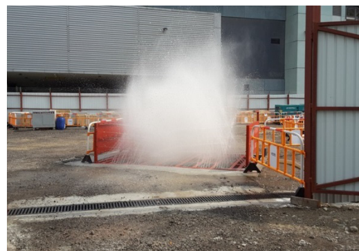
Installation of wheel washing facilities at stockpiling area
