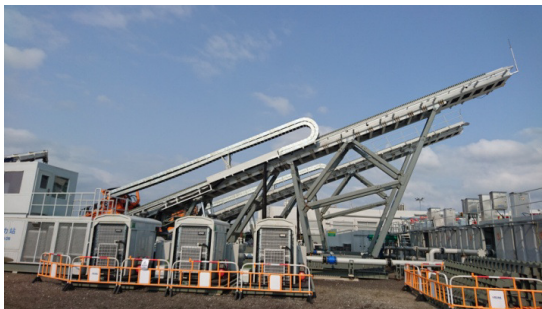
Installation of HDD plants at HDD launching site
