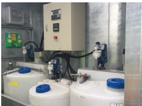
Installation of wastewater treatment facilities at HDD launching site
