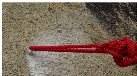
Installation of safe access facilities around the daylighting location on Sheung Sha Chau Island
