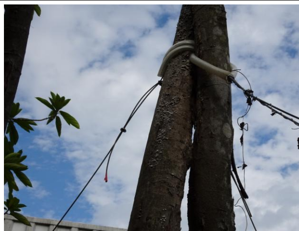
Photo 10. Fungal attack on TA572
