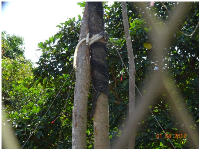
Photo13. A section of TA572 was wrapped by Shelter (遮光網)
