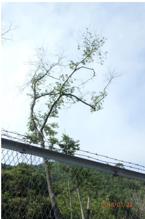
Photo 8. Weak crown of TA327
