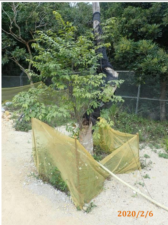
Photo 11. No equipment, waste, or construction materials shall enter the plant protection zone. Collapsed fence shall be promptly rectified.
