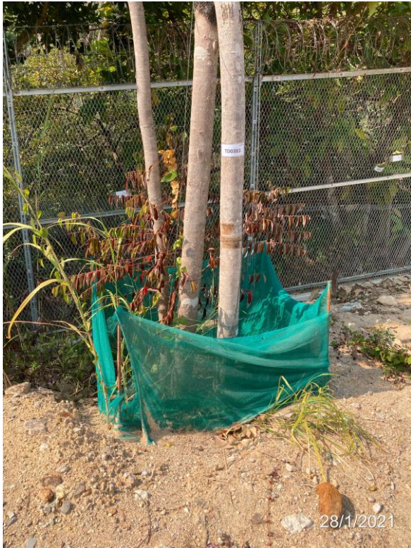
Photo 9. Collapsed fencing to be rectified
