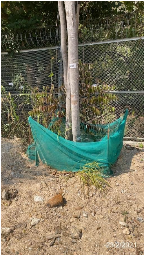
Photo 9. Collapsed fencing to be rectified
