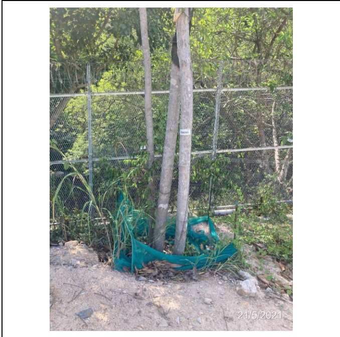
Photo 8. Collapsed fencing of TA572 to be rectified
