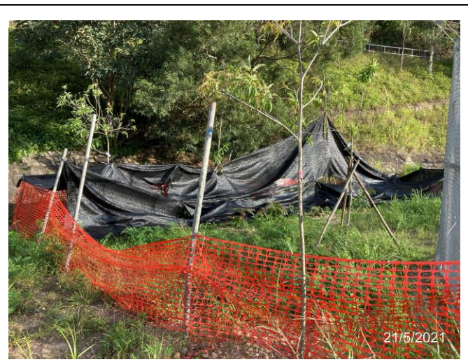
Photo 2. Collapsed shelter for Cibotium barometz to be rectified
