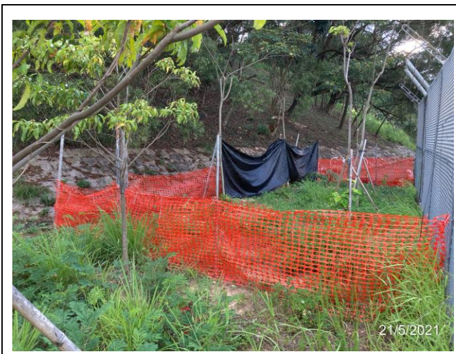
Photo 1. Collapsed shelter for Cibotium barometz to be rectified
