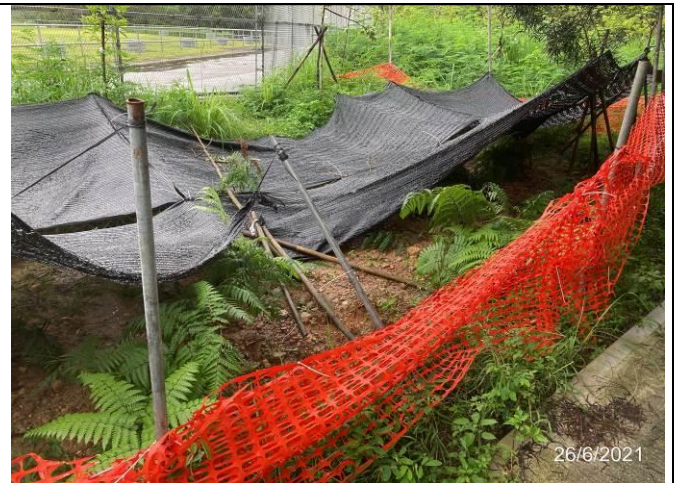
Photo 2. Collapsed shelter for Cibotium barometz to be rectified
