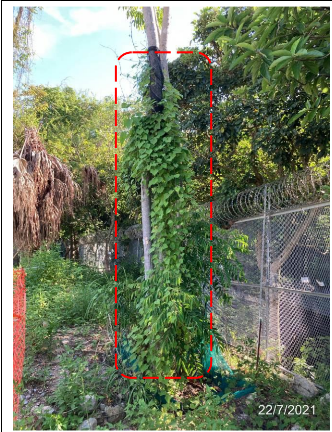
Photo 10. Collapsed fencing of TA572 to be rectified. The climbers on trunk shall be cleared.
