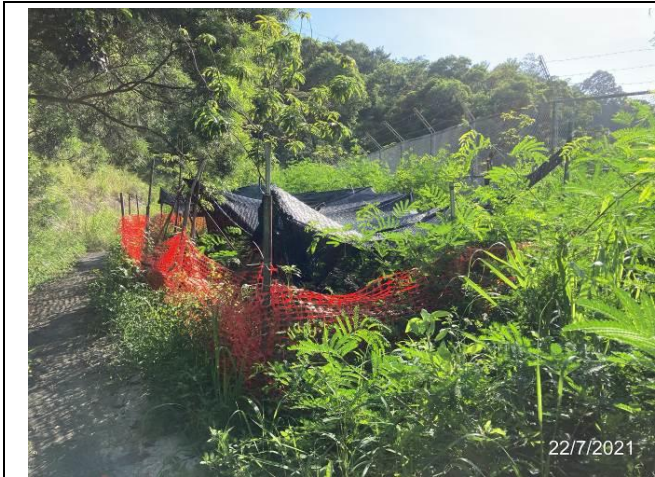
Photo 1. Excessive grass and invasive trees shall be removed properly.
