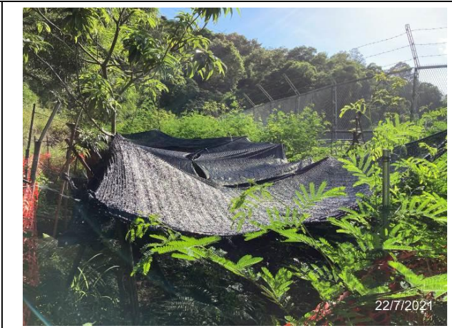
Photo 2. Previously collapsed shelter has been repaired
