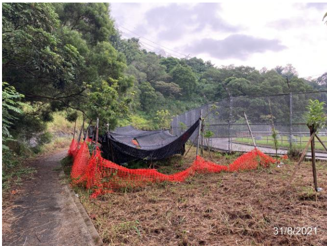
Photo 1. Excessive grass and invasive trees have been removed
