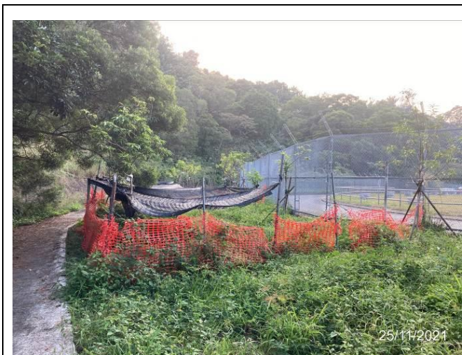
Photo 1. Excessive grass and invasive trees have been removed
