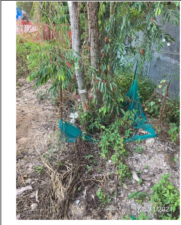
Photo 10. Collapsed fencing to be rectified. The climbers and weeds have been cleared.
