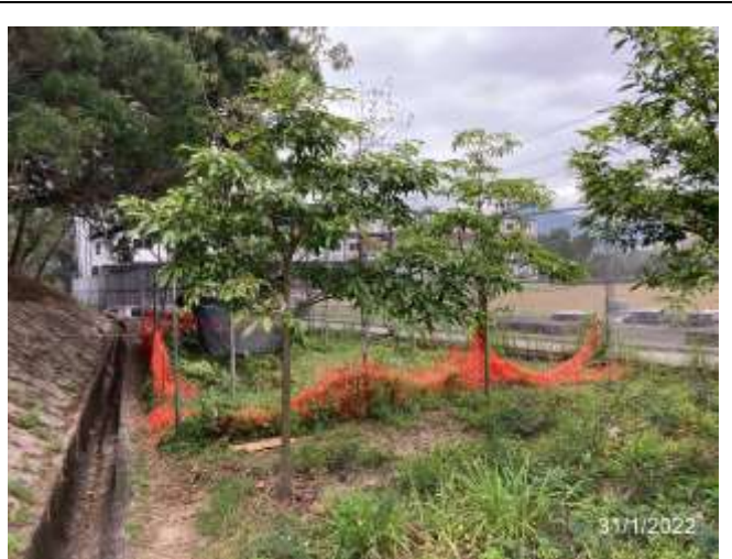
Photo 2. Broken fencing to be rectified
