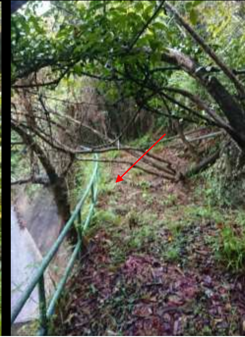
Photo 5 (M1, Slope opposite to project site)
