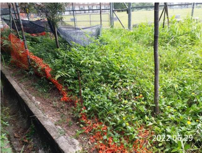
Photo 5. Collapsed shelter to be rectified to cover the exposed Cibotium barometz
