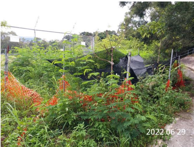
Photo 3. Broken fencing to be rectified
