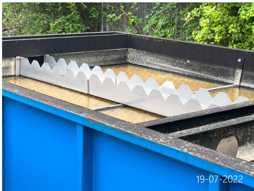
Photo 2 (Water tank at 6/WSD)
