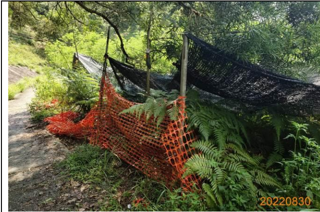
Photo 1. Broken orange fencing to be rectified
