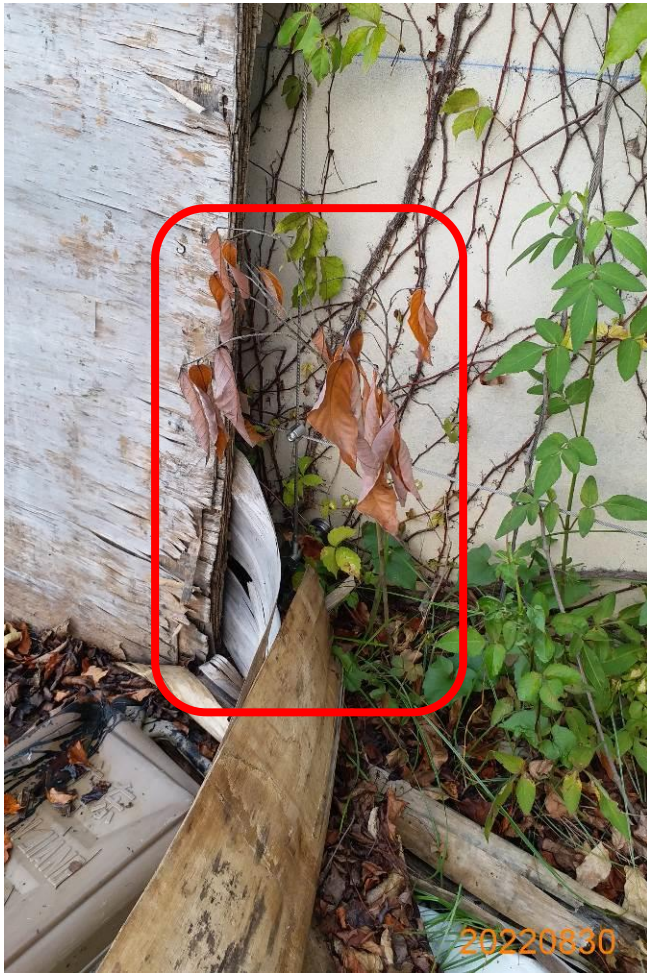
Photo 10. Desmos chinensis is dying if not dead. Construction materials shall be taken away to avoid soil compaction and potential disturbance to the plant.
