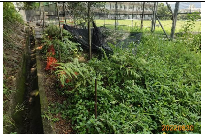
Photo 6. Collapsed black shelter to be rectified to cover the exposed Cibotium barometz
