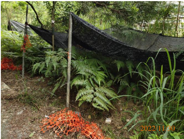
Photo 1. Broken orange fencing to be rectified
