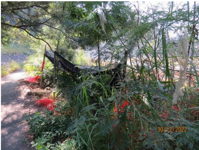
Photo 1. Broken orange fencing to be rectified
