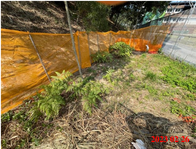
Photo 3. Garbage was cleared out of the protection zone
