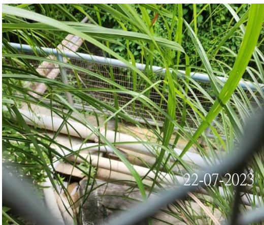
Photo 3 (Discharge point at 6/WSD)
