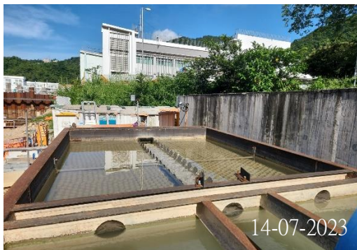
Photo 2 (Water quality of water treatment tank at 6/WSD)
