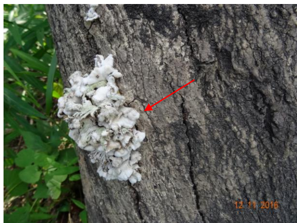
Photo 10. A fungi was observed on tree basement of TA327
