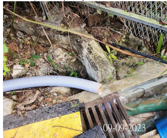
Photo 4 (Discharge point at 6/WSD)
