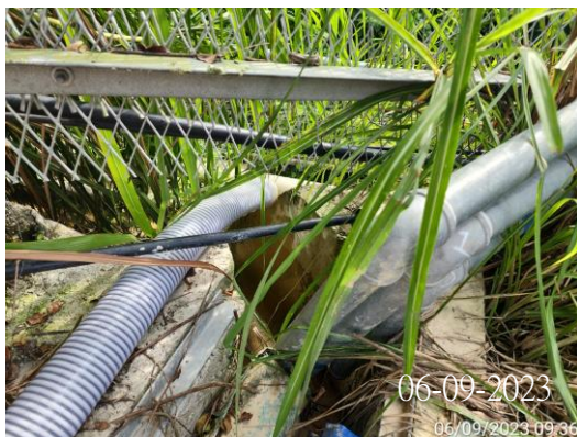
Photo 3 (Discharge point at 6/WSD)
