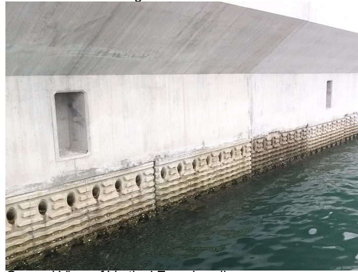
General View of Vertical Eco-shoreline
