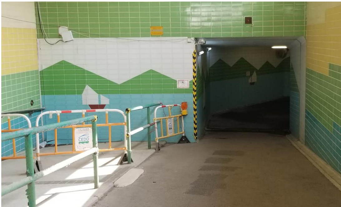
Photo 3 - Erection of site hoardings in unobtrusive colours
