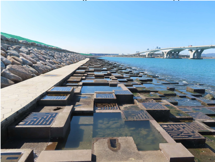
General View of Rocky Eco-shoreline
