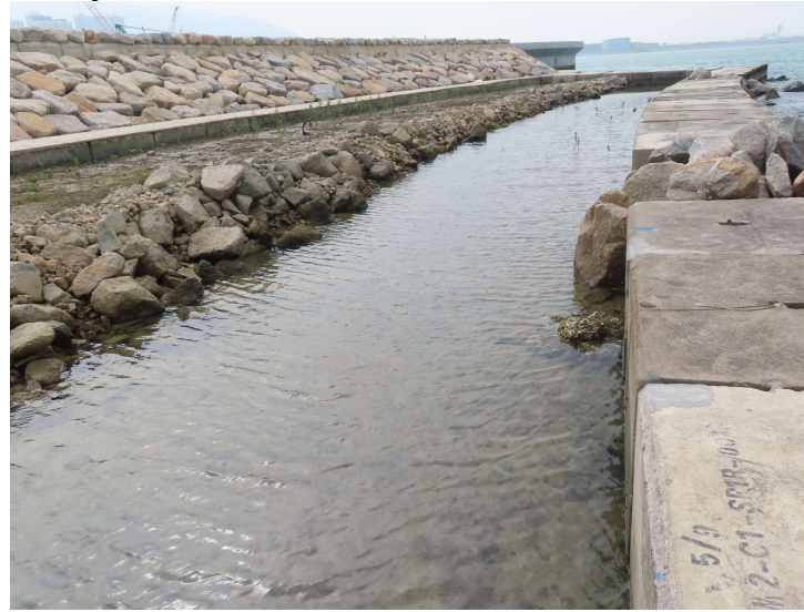
General View of Mangrove Eco-shoreline at Lower Terrace
