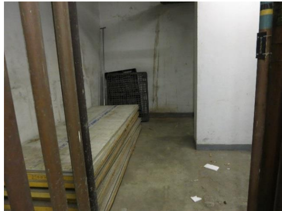
Figure 3.14 Panels stored in the Incinerator Room
