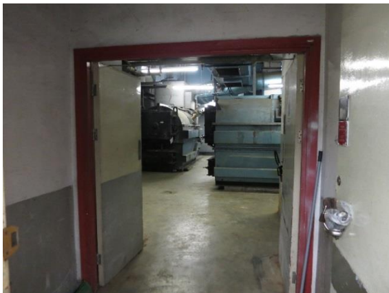
Figure 3.1 Entry Hallway of Incinerator Room
