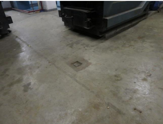
Figure 3.13 Sealed Drain at the Incinerator Room
