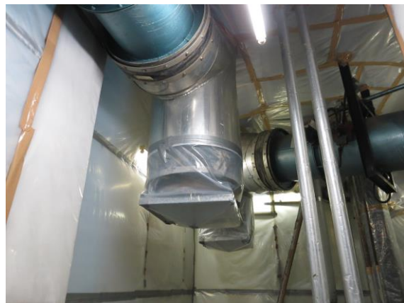
Figure 3.2 Chimneys sealed with fire retardant polythene sheets
