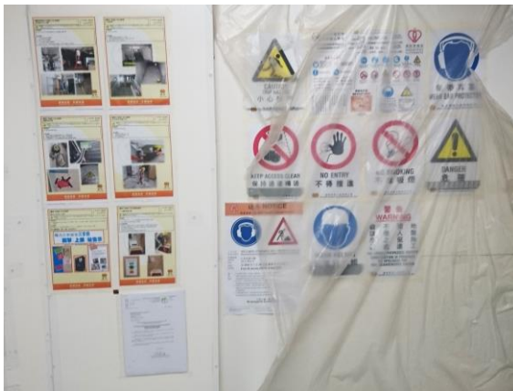
Figure 3.11 Environmental and Safety Notices and Warning Signs were posted in the entry of Incinerator Room
