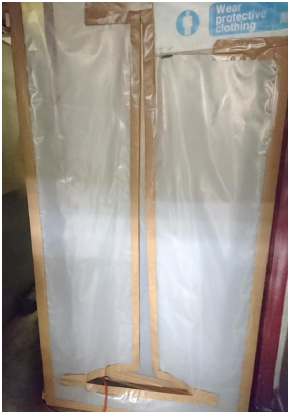
Figure 3.5 Three-compartment decontamination unit for entry and exit into the works area
