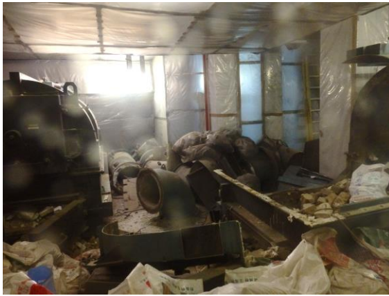
Figure 3.2 View of Incinerator Room
