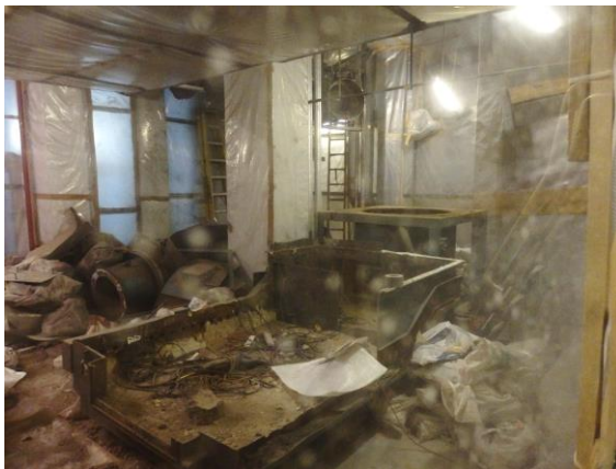
Figure 3.3 Demolition of Incinerator No.2
