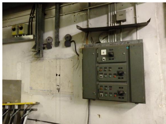
Figure 3.8 Wall-mounted control panel for incinerators was demolished
