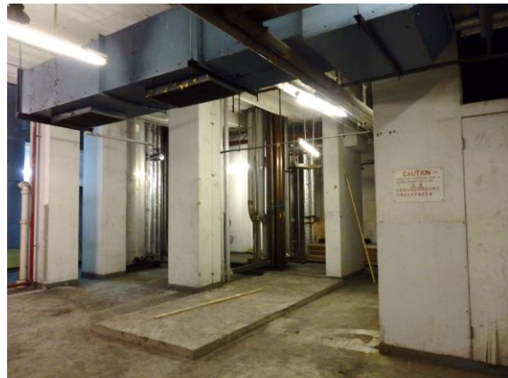
Figure 3.6 Demolition of Incinerator No.2 was completed
