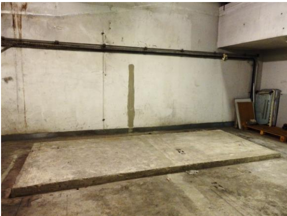
Figure 3.5 Demolition of Incinerator No.1 was completed
