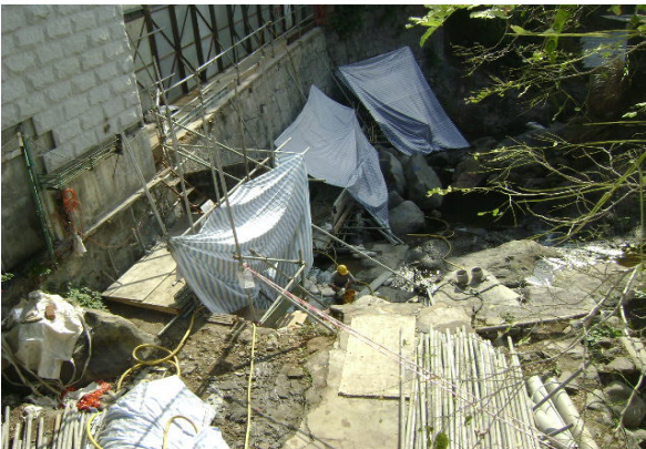
Construction activities at I-2-C
