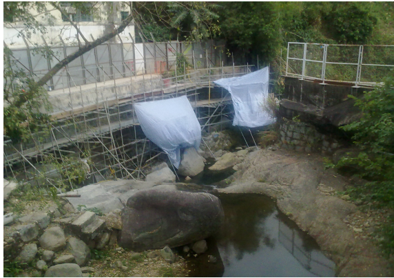
Construction activities at I-2-C.
