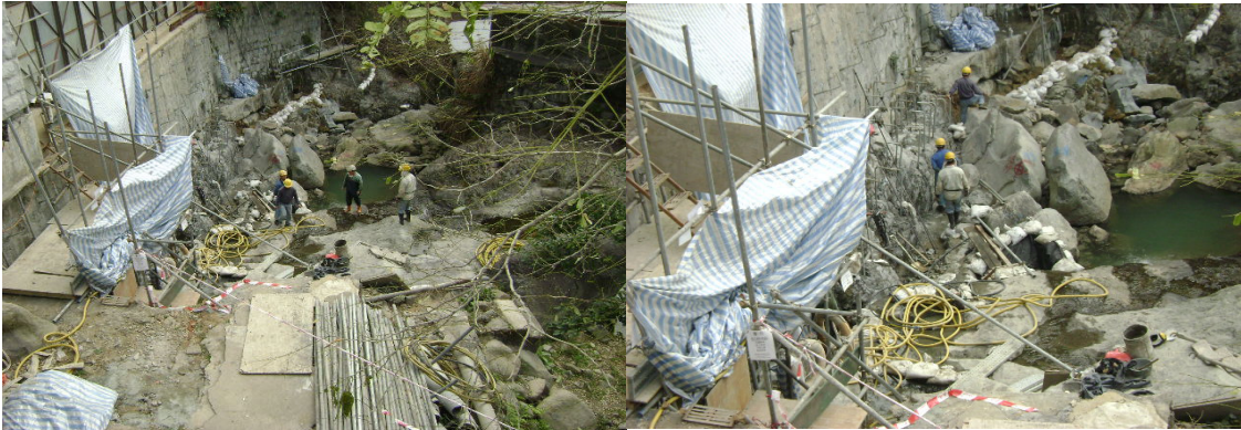
Construction activities at I-2-C
