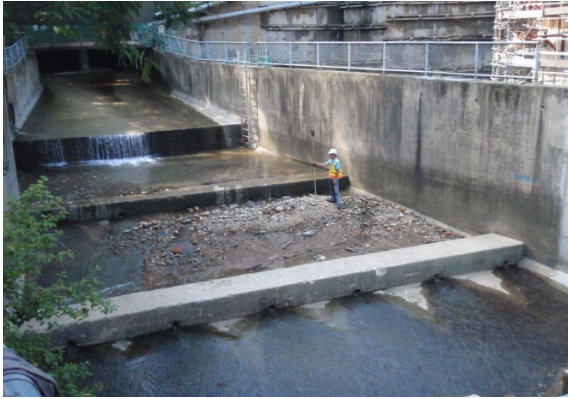
Site photo. As advised by Contractor, rocks and soil were found washed down to the stream from the upstream
