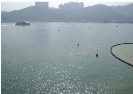
A photo showing slit curtain was functioning properly to prevent suspended solids dispersed away from the site
