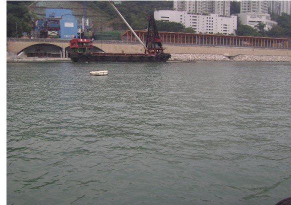
Photographic record for exceedance of Dissolved Oxygen (marine surface) recorded at O-1(FT) on 14-Dec-11
