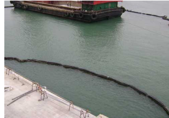
Photographic record for exceedance of Dissolved Oxygen (marine surface) recorded at O-1(FT) on 09-Dec-11
