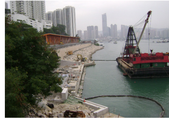
Photographic record for exceedance of Dissolved Oxygen (marine surface) recorded at O-1(FT) on 05-Dec-11
