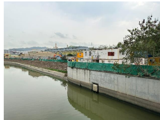
Construction Activities (Ng Tung River) (Non-Project-related, taken on 28 Mar 2024)
