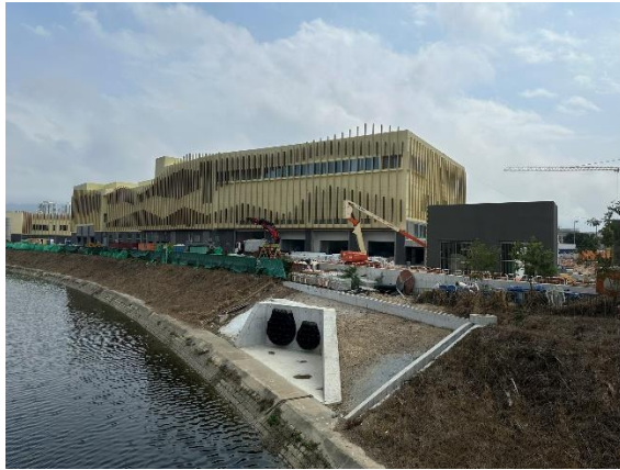
Construction Activities (Ng Tung River) (Project-related, taken on 4 Mar 2024)
