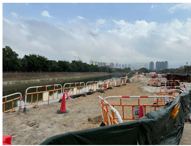
Construction Activities (Sheung Yue River) (Non-project-related, taken on 4 Mar 2024)
