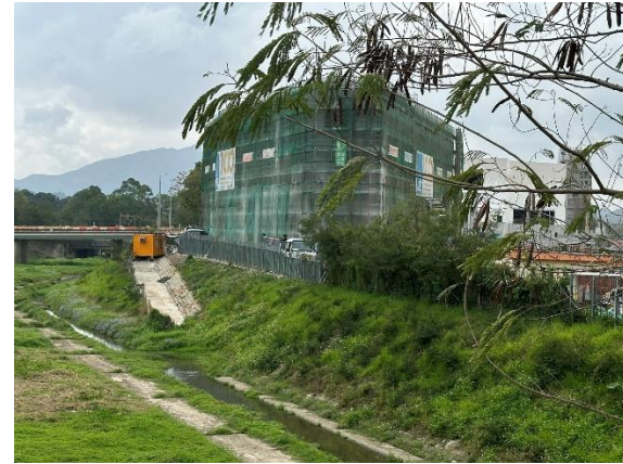
Construction Activities (Shek Sheung River) (Project-related, taken on 12 Mar 2024)
