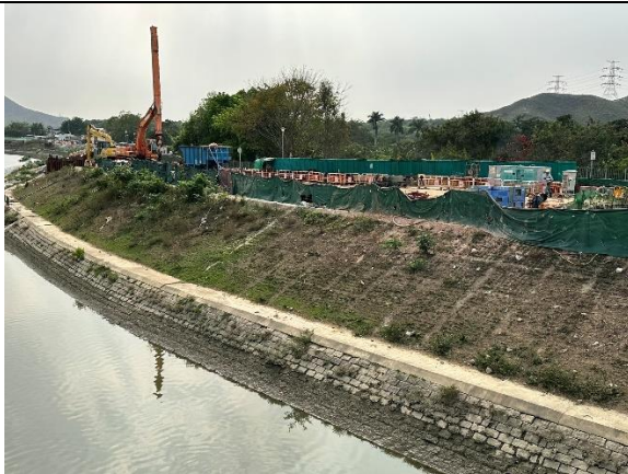
Construction Activities (Sheung Yue River) (Non-project-related, taken on 21 Mar 2024)
