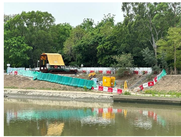
Construction Activities (Sheung Yue River) (Non-project-related, taken on 28 Mar 2024)
