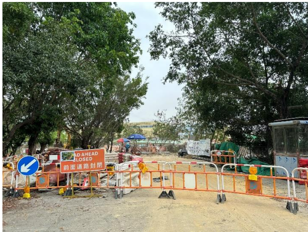
Construction Activities (Ng Tung River) (Non-Project-related, taken on 21 Mar 2023)
