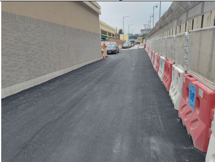
Construction of Temporary Pavement by Asphalt
