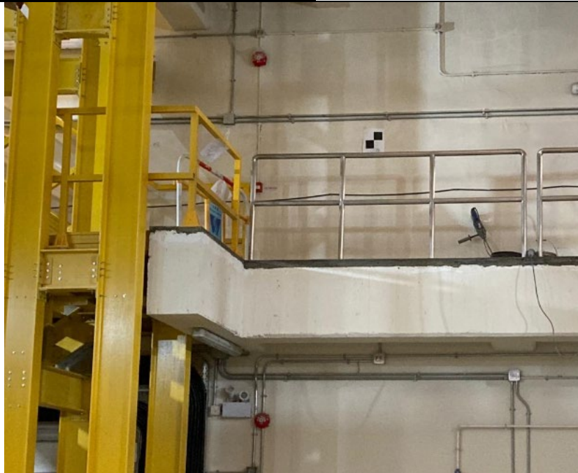
Installation of Railing at ReWPFS
