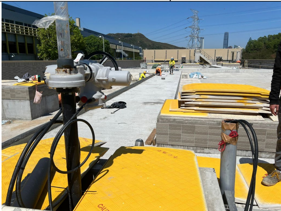
Construction of roof footpath
