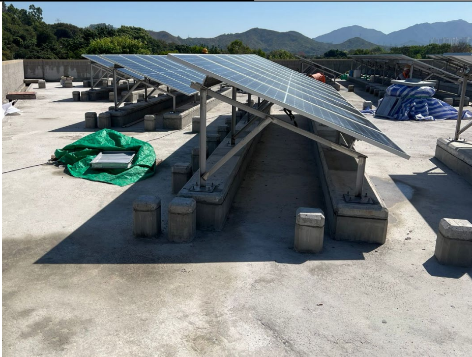
Installation of solar panel
