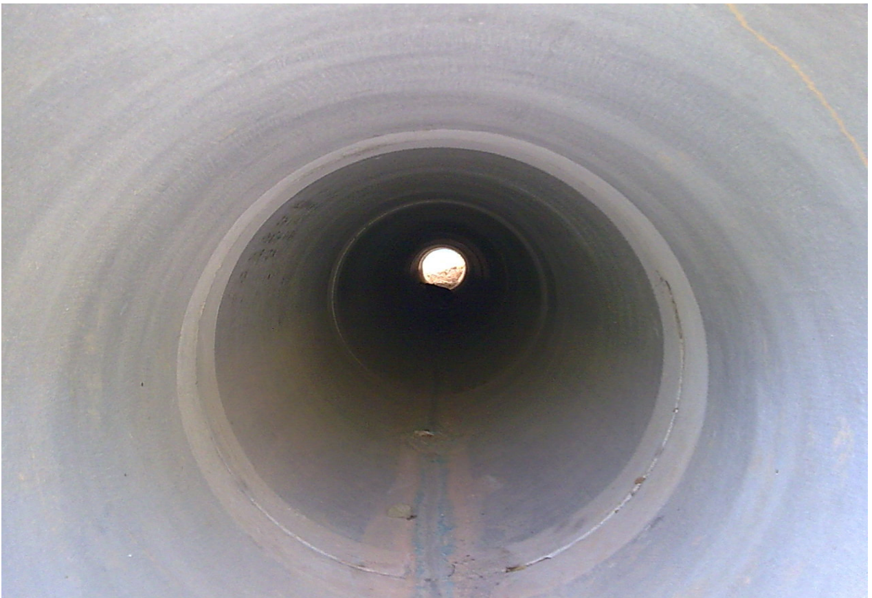
(2) Inside Wildlife Tunnel (C)
