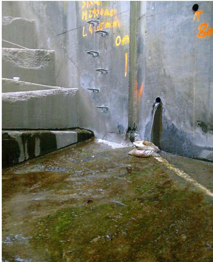
(10) The wall of the Wildlife Tunnel (A)
