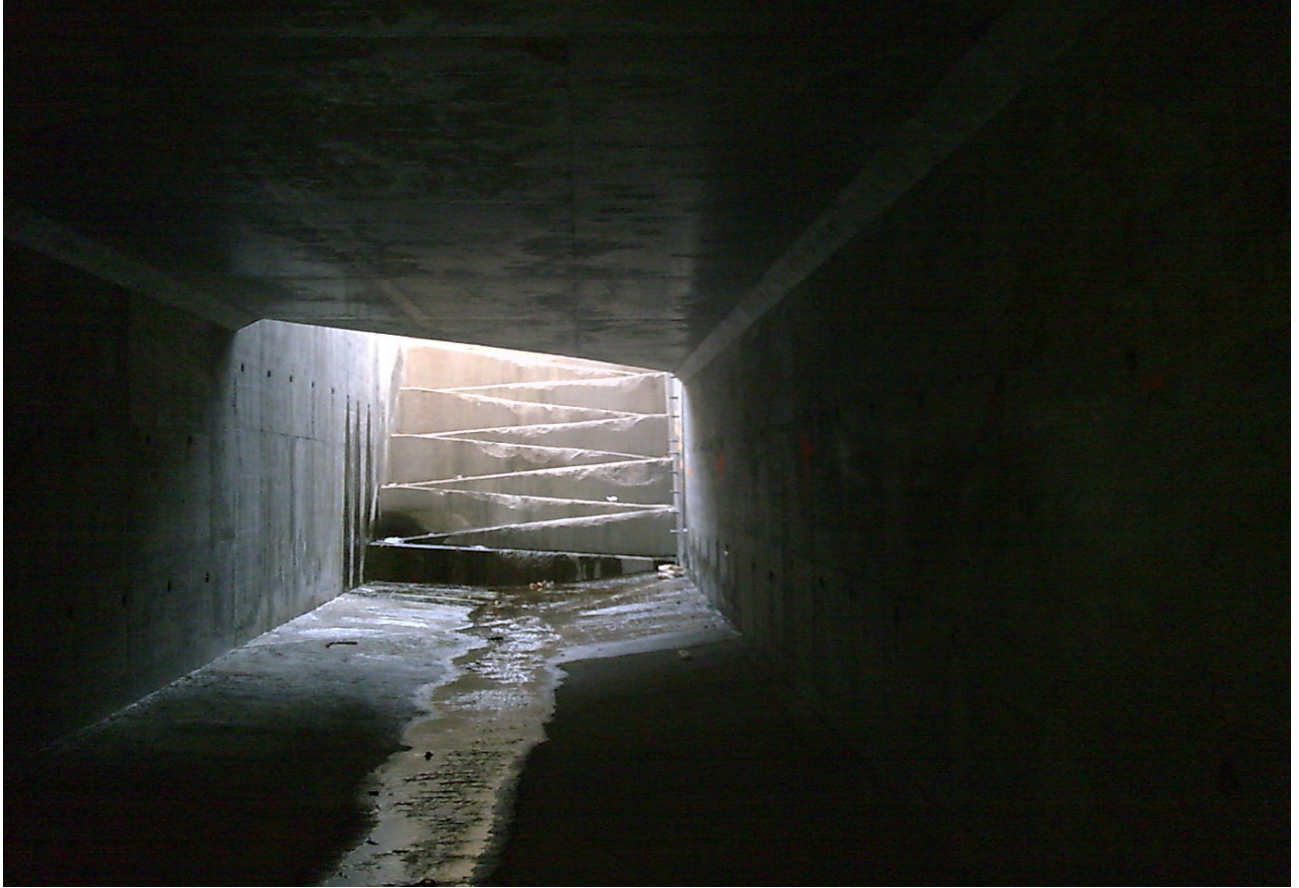
(9) Another view inside the Wildlife Tunnel (A)
