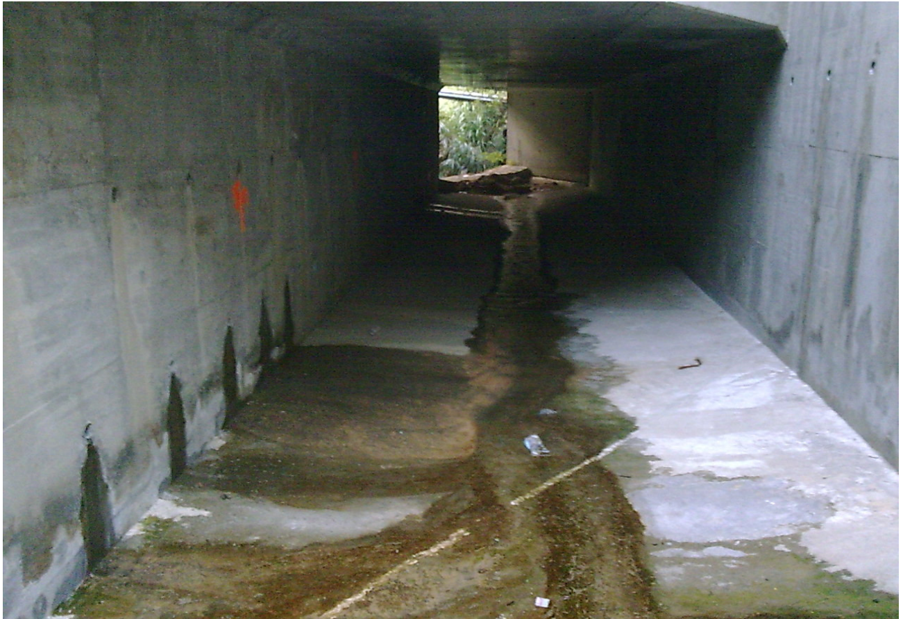
(8) Inside the Wildlife Tunnel (A)
