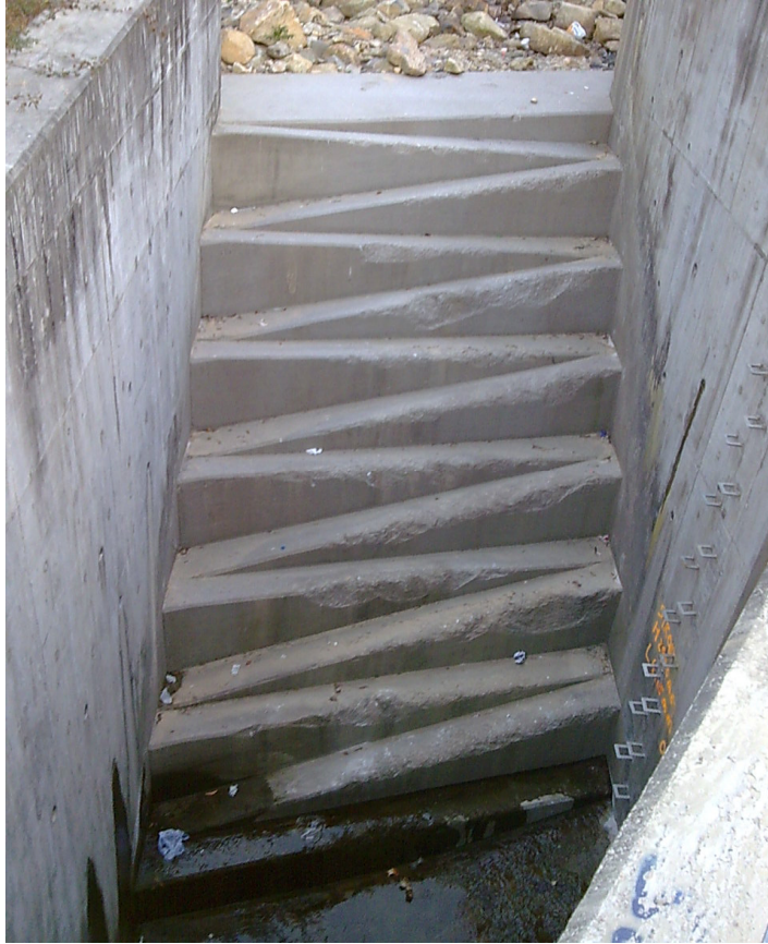
(7) The sloped Step at Wildlife Ramp (A)
