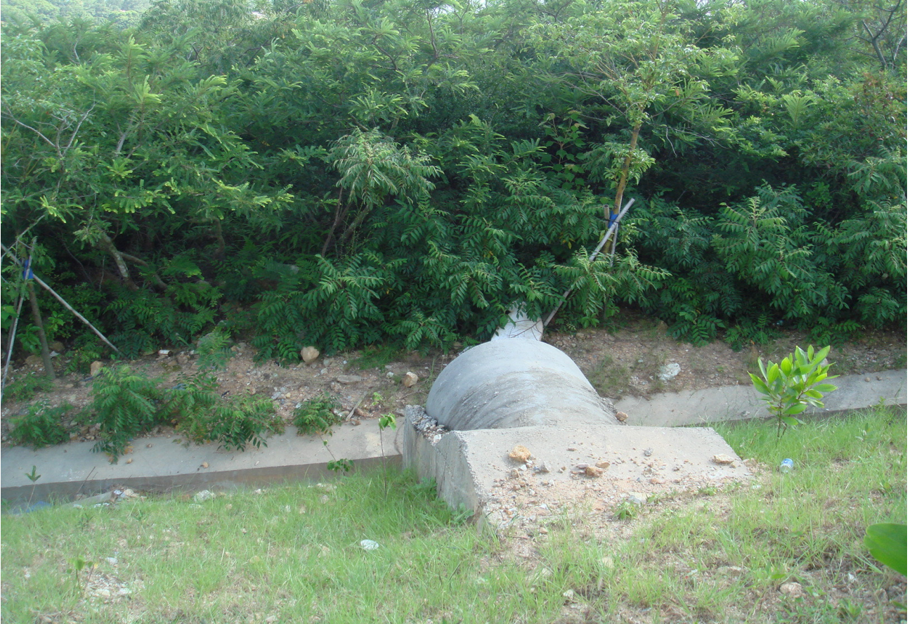
(5) Opening / Entracne of the Wildlife Tunnel (B)
