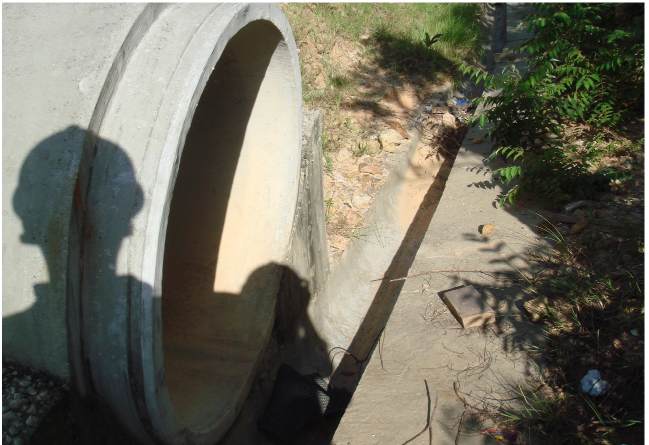
(6) Opening / Entrance of Wildlife Tunnel (B)
