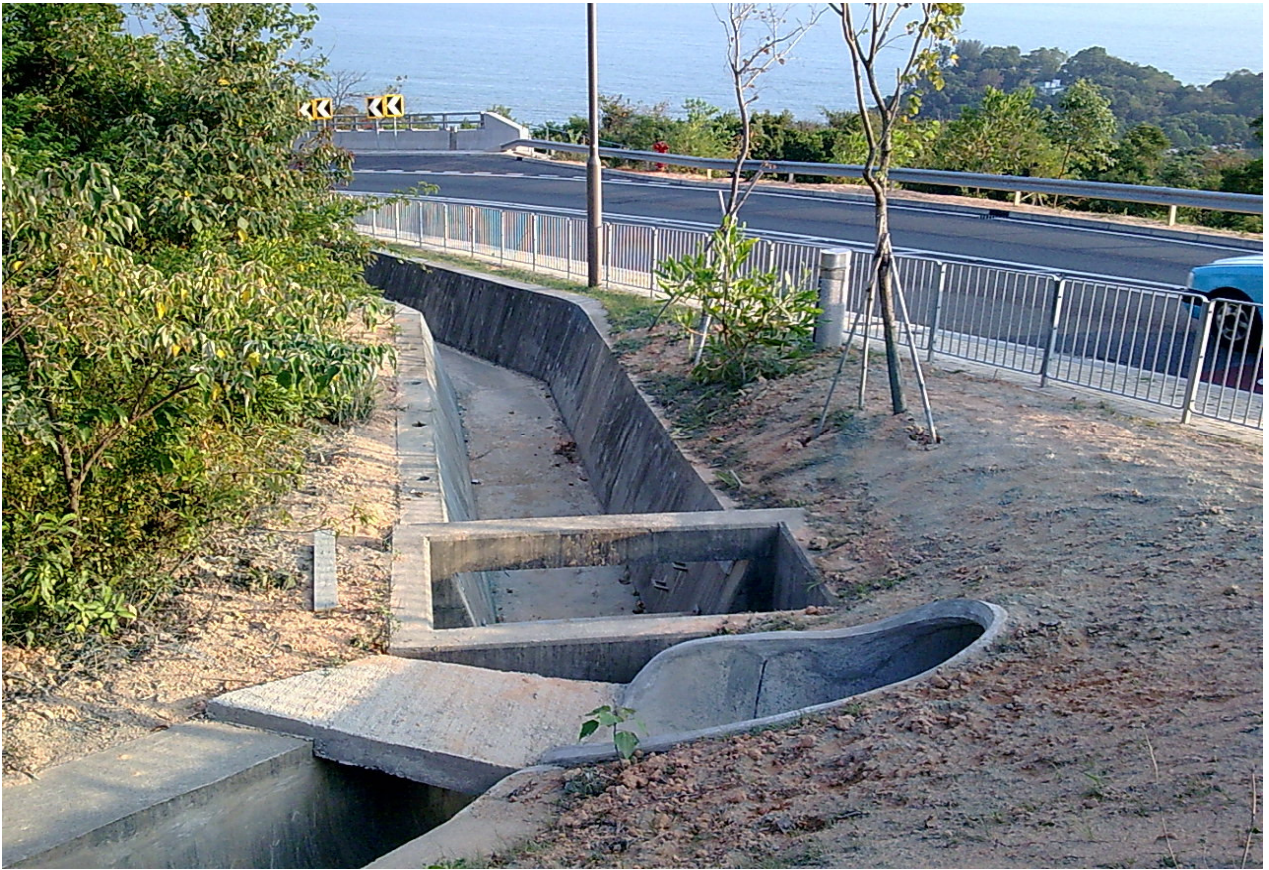
(1) Opening of Wildlife Tunnel (C)
