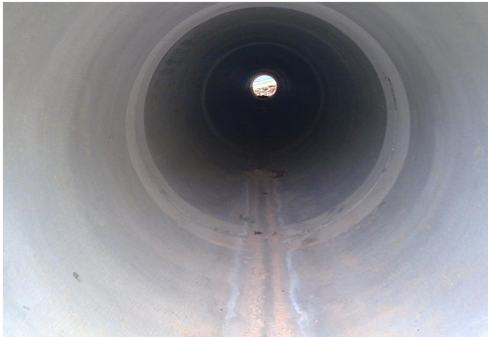
(2) Inside Wildlife Tunnel (C)
