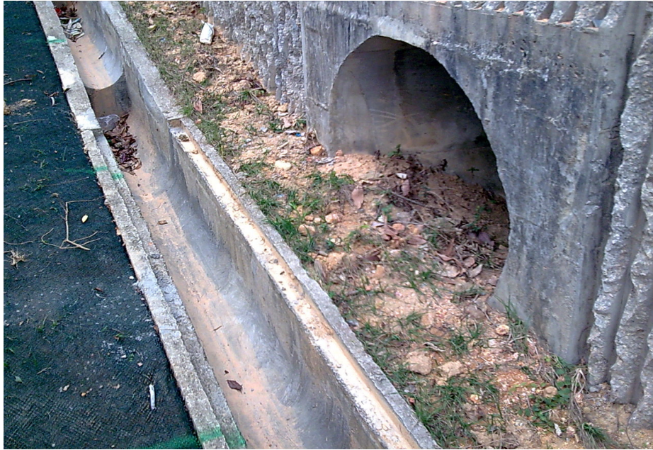
(5) Opening / Entracne of the Wildlife Tunnel (B)
