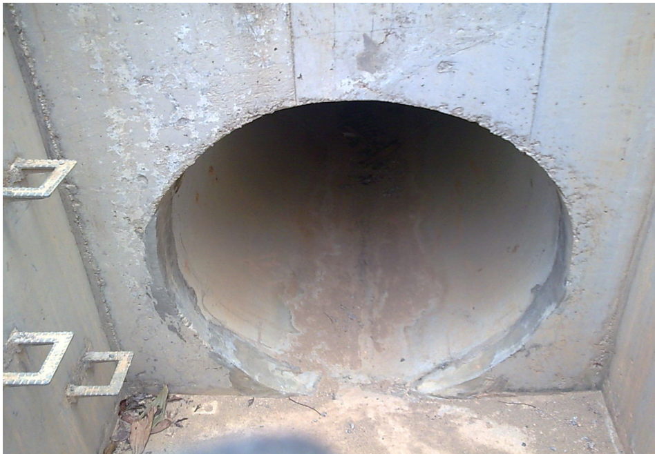
(4) Opening of Wildlife Tunnel (B)
