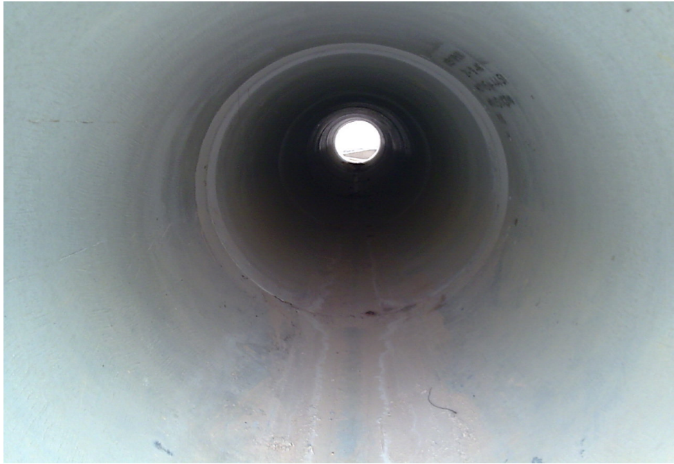
(7) Inside Wildlife Tunnel (B)
