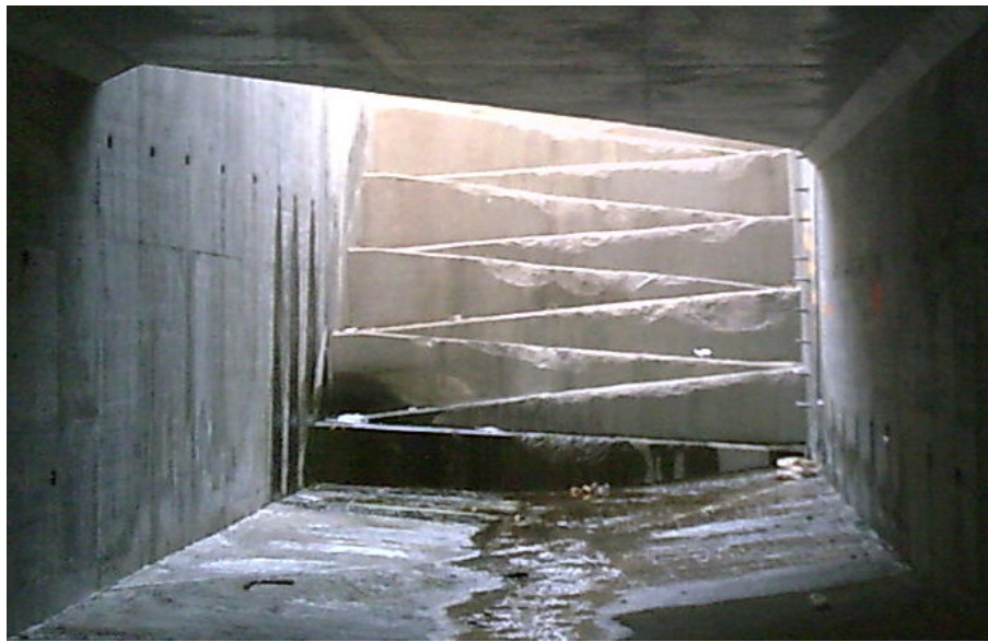
(9) Inside the Wildlife Tunnel (A)
