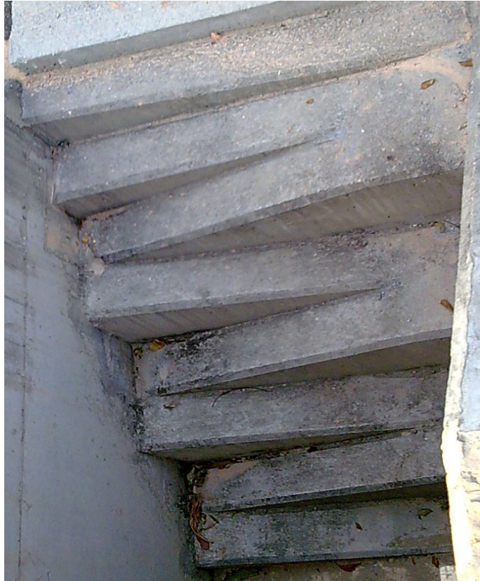
(7) The sloped Step at Wildlife Ramp (A)
