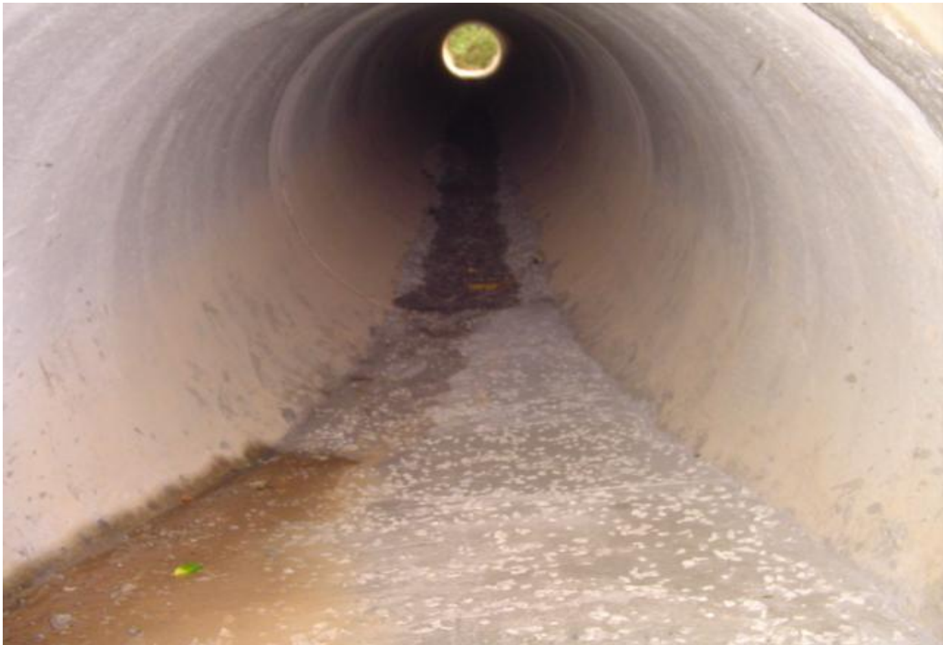
(2) Inside Wildlife Tunnel (C)
