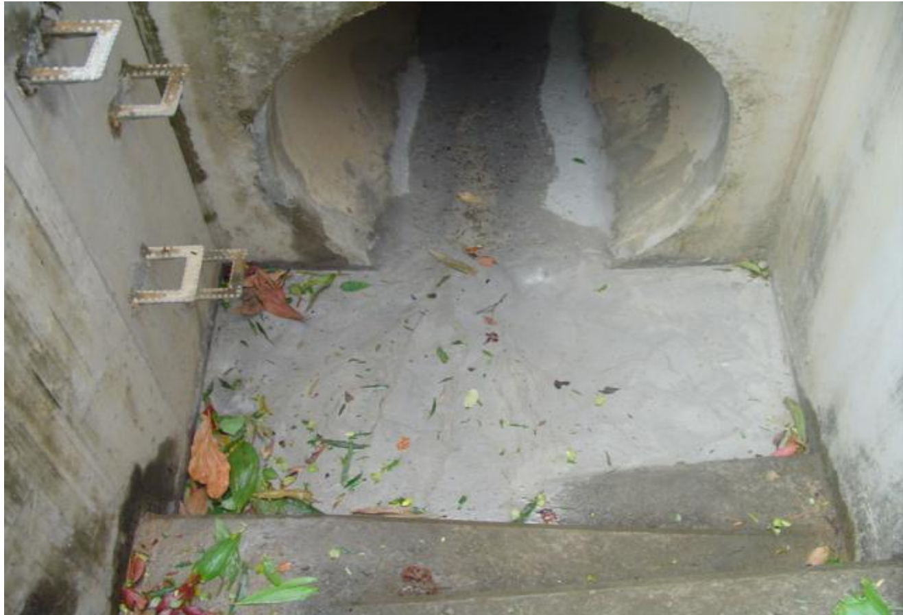
(3) Opening of Wildlife Tunnel with Wildlife Ramp (C)
