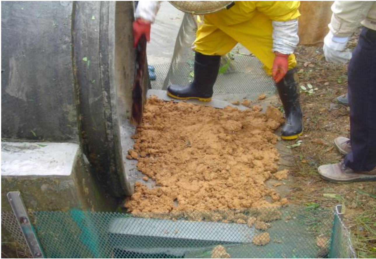
(5) Inside Wildlife Tunnel ( C )
