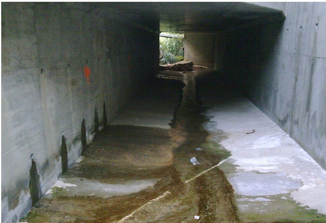
(8) Inside the Wildlife Tunnel (A)
