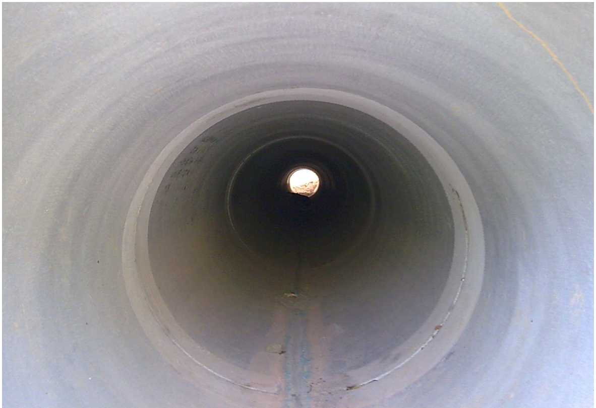
(2) Inside Wildlife Tunnel
