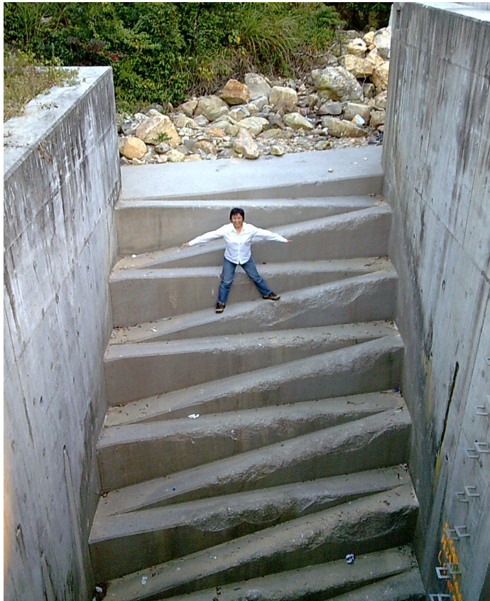
(7) The sloped step at Wildlife Ramp (Stream 15)
