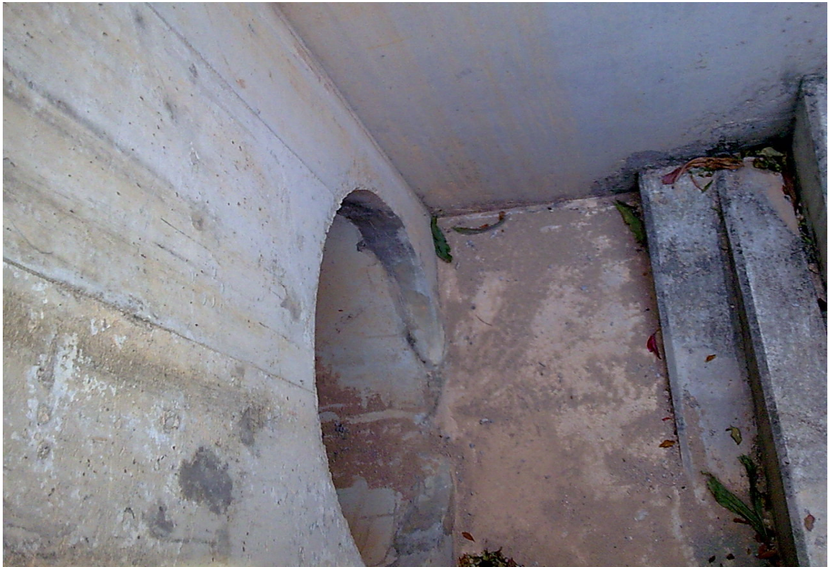
(4) Opening of wildlife tunnel with wilfe ramp
