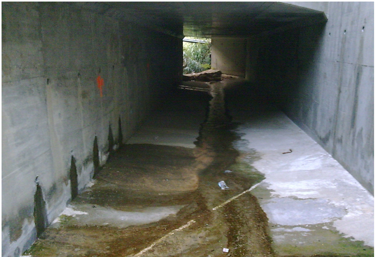
(8) Inside the Wildlife Tunnel(Stream 15)
