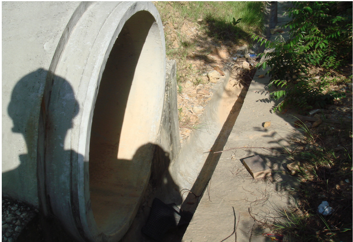
(6) Opening / Entrance of Wildlife Tunnel
