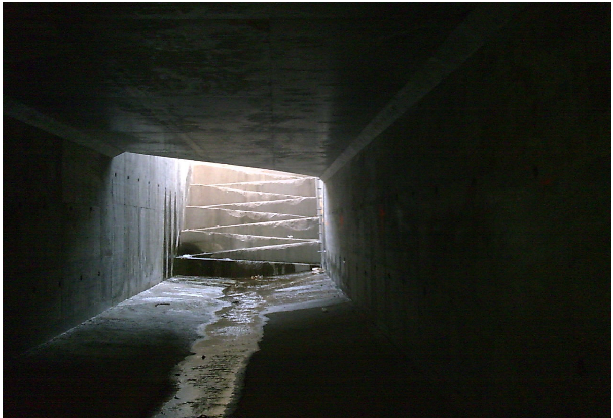
(9) Another view inside the Wildlife Tunnel (Stream 15)
