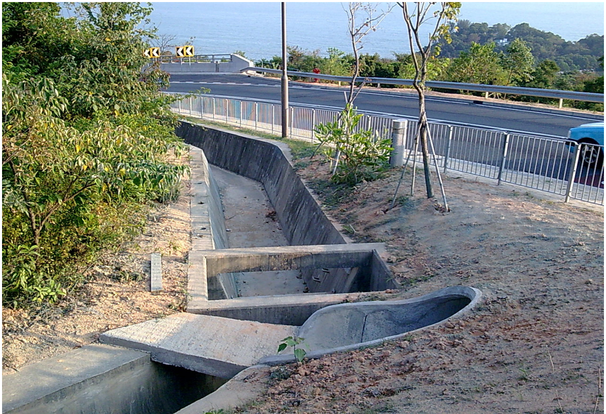
(1) opening of Wildlife Tunnel
