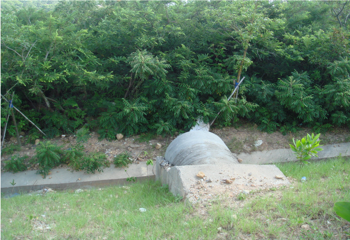
(5) Opening / Entracne of the Wildlife Tunnel
