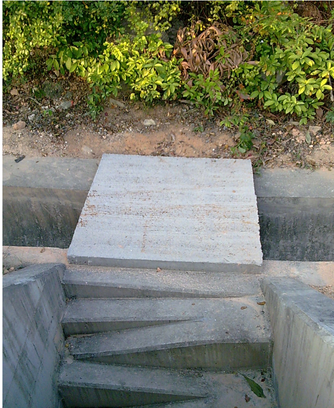
(3) Opening of wildlife tunnel with wilfe ramp
