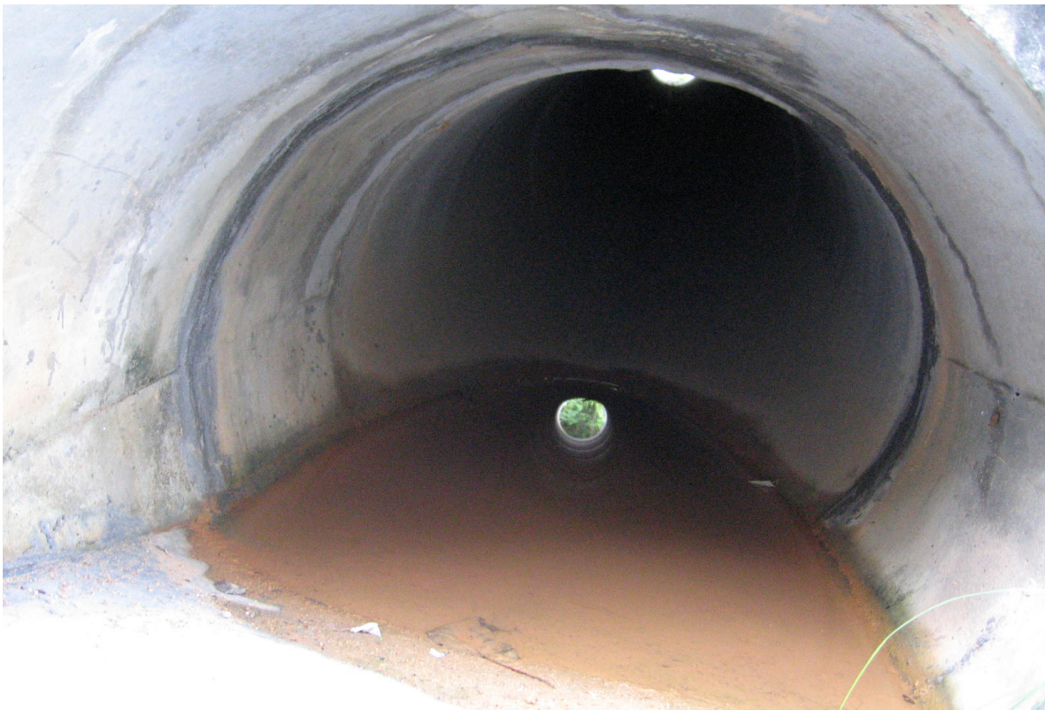
(2) Inside Wildlife Tunnel (C)
