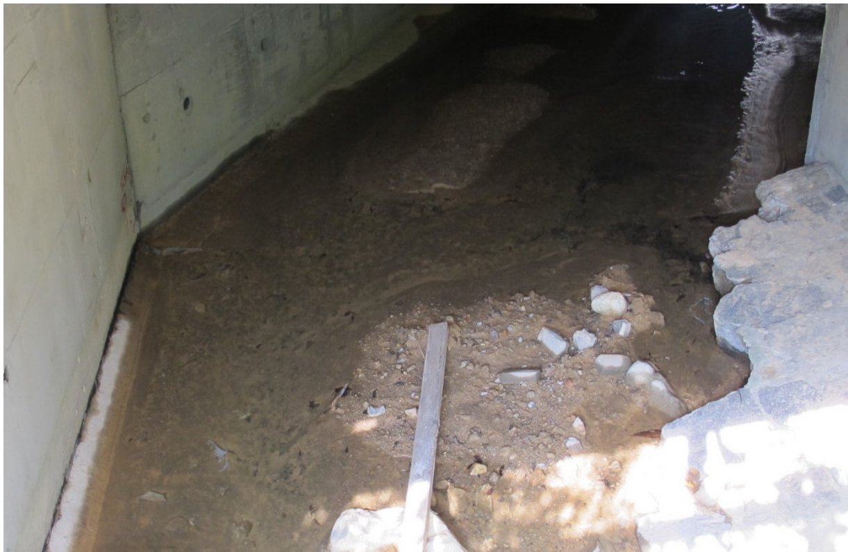
(8) Inside the Wildlife Tunnel (A)
