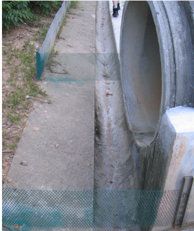
(5) Inside Wildlife Tunnel ( C )
