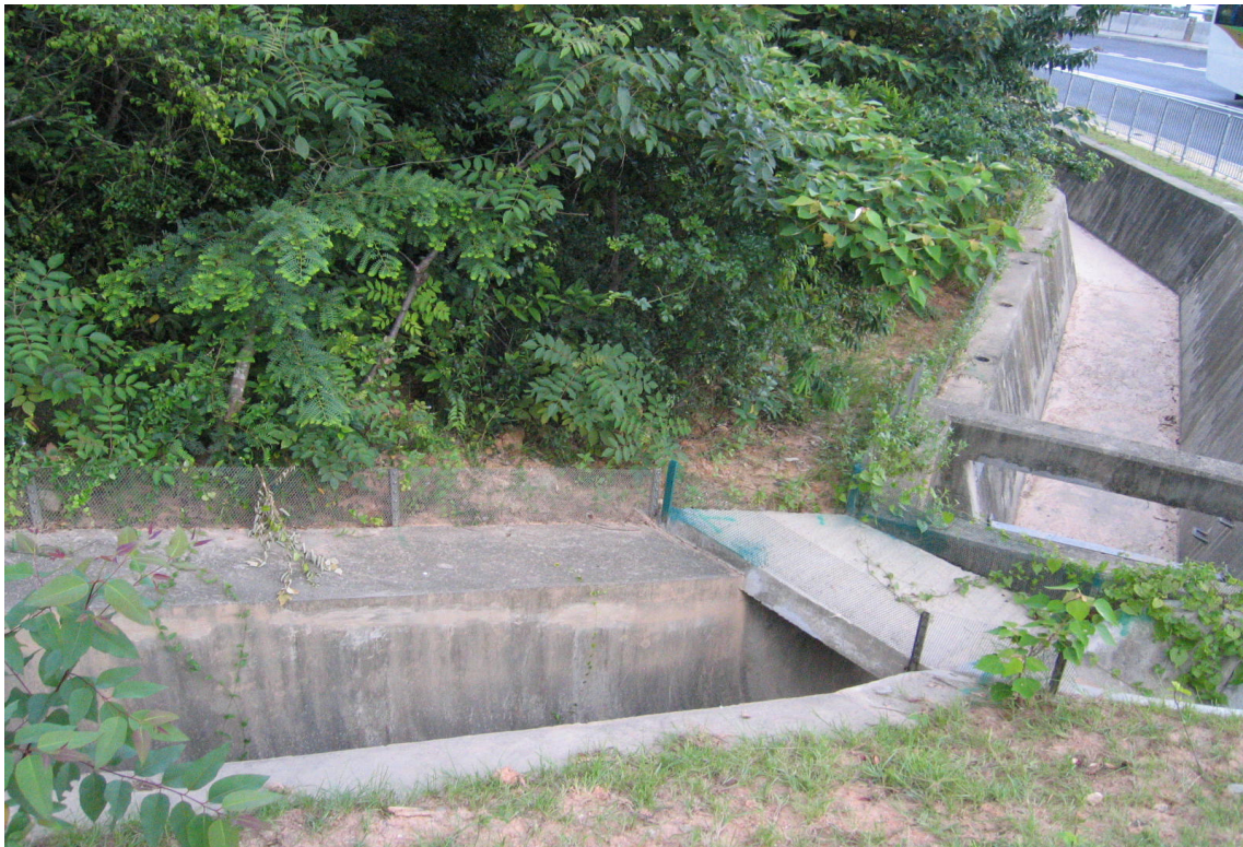
(6) Opening of the Wildlife Tunnel (C)
