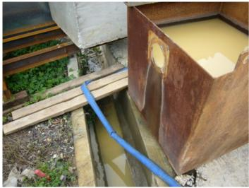
Muddy water discharge into the drainage channel from the sedimentation tank was observed at CH290. The Contractor was reminded to stop the discharge and provide the effective sedimentation or improved the desilting system efficiency before any discharge was undertaken.
