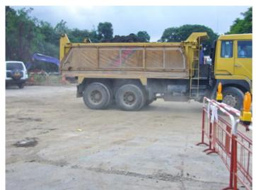
Obs 1 – Fugitive dust emission from the site was observed at CH290 during the site inspection, the Contractor was reminded to provide water spraying or implement the dust suppression on necessary basis.
