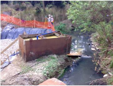
Muddy water discharge from the sedimentation tank was observed at CH200, the Contractor was reminded to improve the desilting system in effective/efficiency condition.
